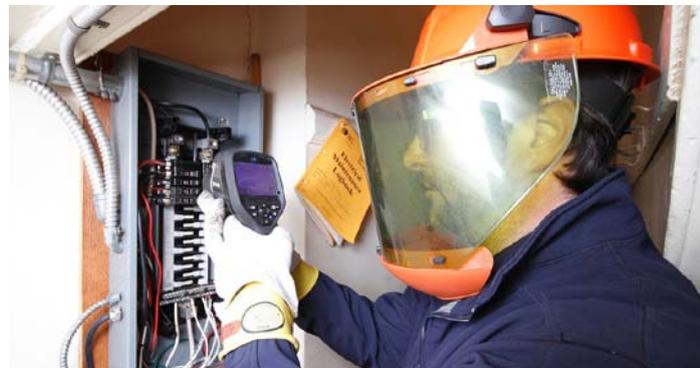
Innovative technology, like speciality infrared scanners, is used to inspect the electrical panel in older homes.
